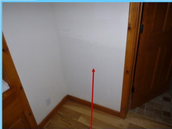
Previous drywall patch on backside of bathroom plumbing wall.
