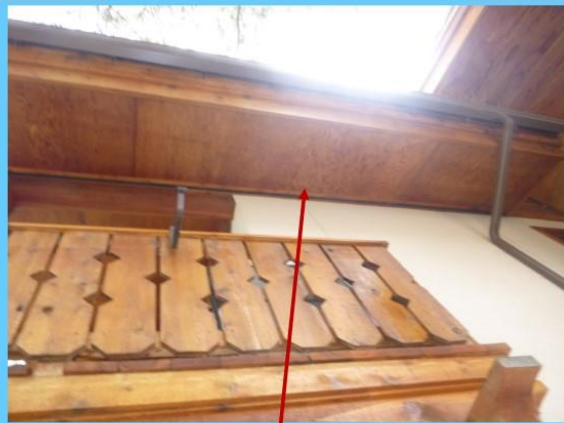
Soffit venting to the roof system.
