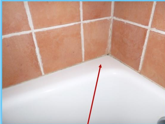
Missing/cracked grout.
